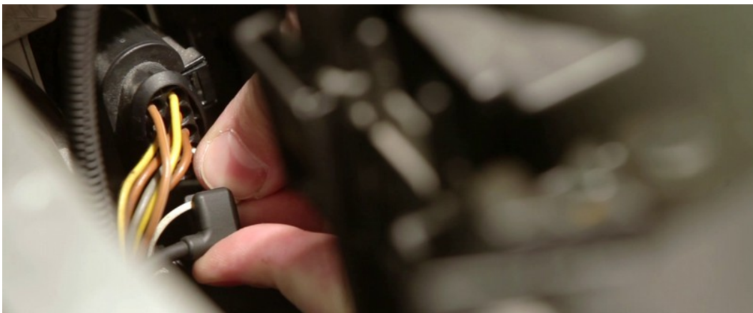
Fig 9. Installation of the current sensor on original high beam cable.
